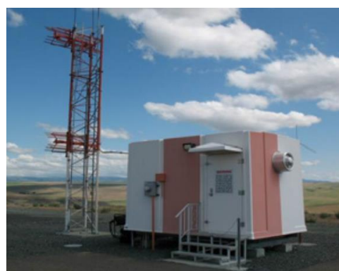
Typical Glide Slope Antenna (FAA)
