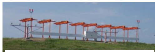
Typical Localizer Antenna Array (FAA)
