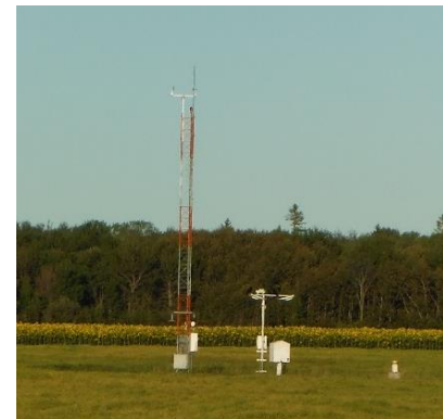
Typical Weather Reporting Station System
