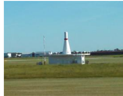
Minot VOR Facility
