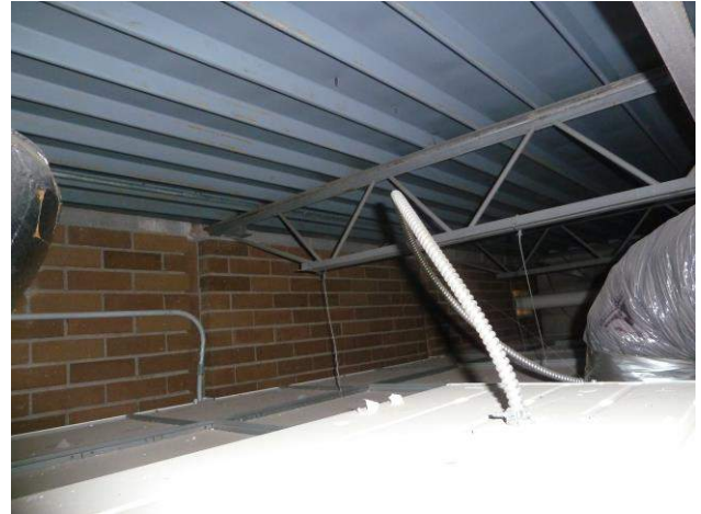
Photo #14: East living quarters addition – roof joists bearing on east wall of original building.
