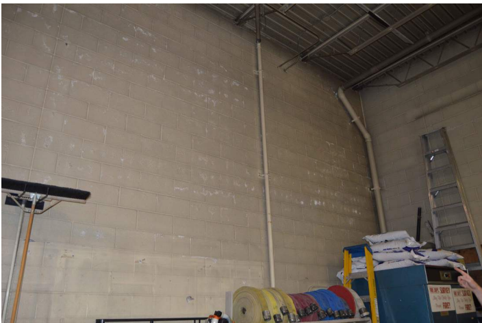
Apparatus Bay #1 - Efflorescence on North Wall
