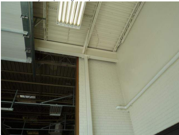
Photo #17: NE corner of original building apparatus bay, viewing 2011 steel column and beam line at west side of bay extension addition (Looking West)
