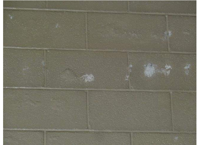
Photo #9: close up of spalling and white Efflorescence at north wall of 1978 addition.
